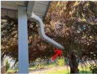
**Attention Needed-** The gutters on the rear of the home appear to have rusted through and need to be replaced.
