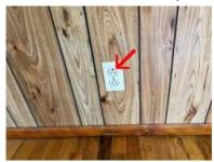
The noted outlet has the hot and neutral wires reversed. Note-Any outlets with cracked ground
