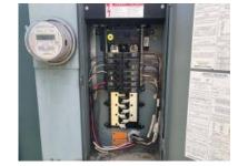
Condition of Wiring in Panel: Satisfactory - Electrical circuitry wiring in the panel appears neatly arranged with no
